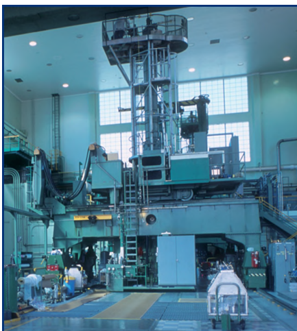
The NRU reactor is one of the most versatile research reactors in the world which also provided the knowledge required for the development, maintenance and evolution of the fleet of CANDU nuclear reactors in Canada.
