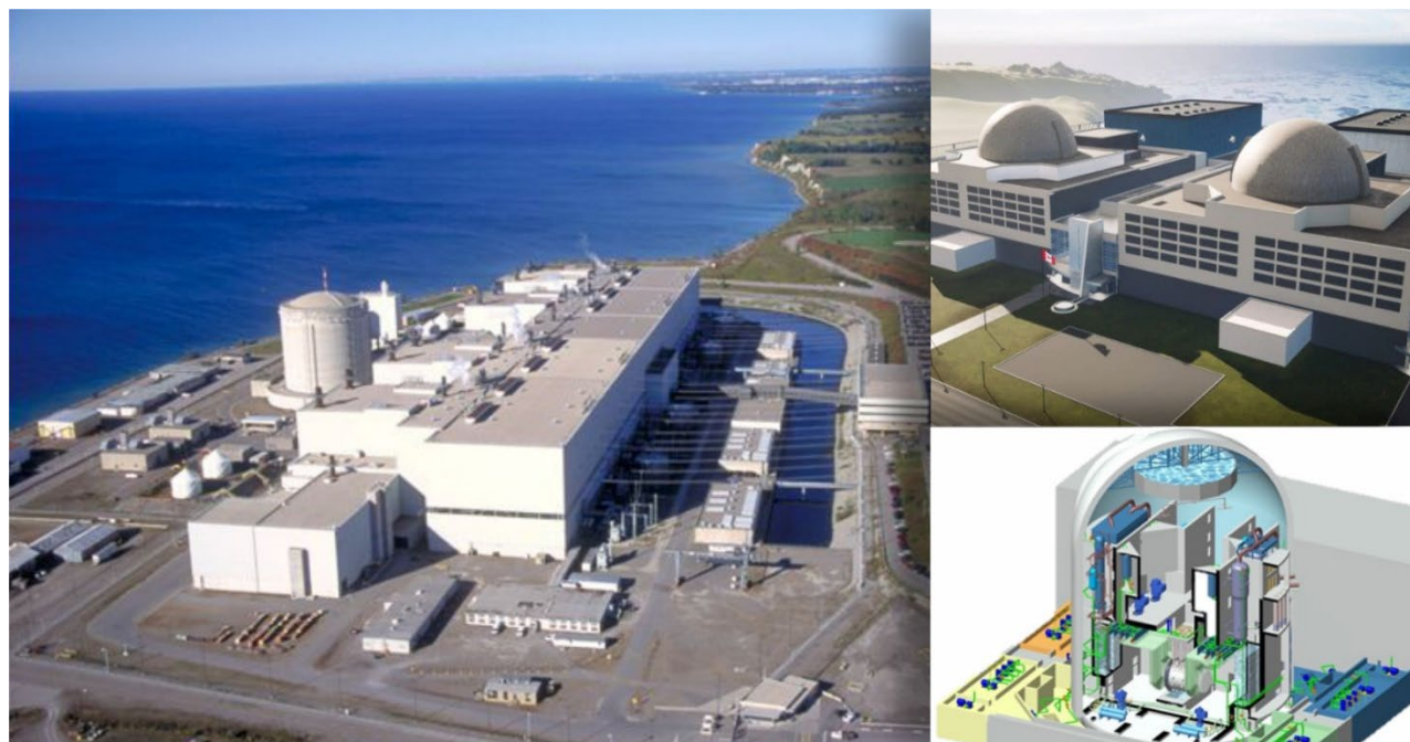
Figure 11. Darlington NPP near Toronto (3600 MW from four CANDU units). (Photo source: OPG) Inset right: CANDU MONARK (1000 MW, developed by AtkinsRéalis - Candu Energy) takes the CANDU product forward, building on over 60 years of fleet experience. (Photo source: AtkinsRéalis - Candu Energy)
