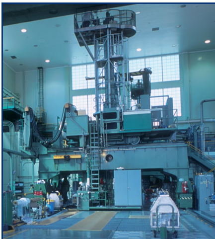
The NRU reactor is one of the most versatile research reactors in the world which also provided the knowledge required for the development, maintenance and evolution of the fleet of CANDU nuclear reactors in Canada.
