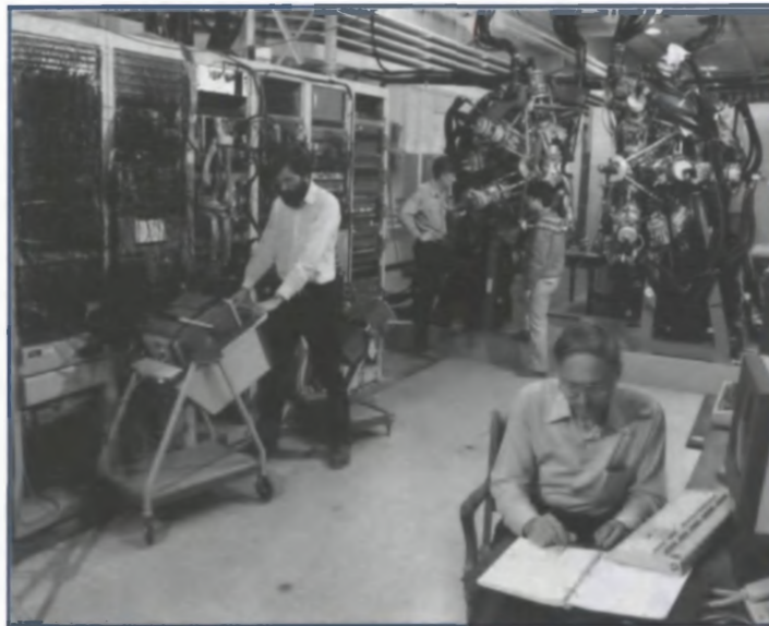
Fig. 2 This 1987 photograph shows the 8 \pi spectrometer at the temporary location it occupied in Target Room 2 prior to the funding of Phase 2 (completion of work on two new target rooms and installation of the beam lines) of the TASCC project. Paul Taras (University of Montreal) is seated at the data acquisition computer terminal and David Radford is looking into the oscilloscope on the left. David Ward (left) is touching the spectrometer, open for target inspection, with Xuan Tran, a technologist from McMaster University, looking on.
